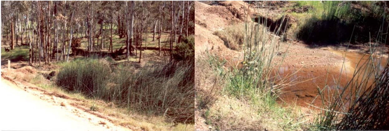
Figure 4.2a. Photos of Site 2.
