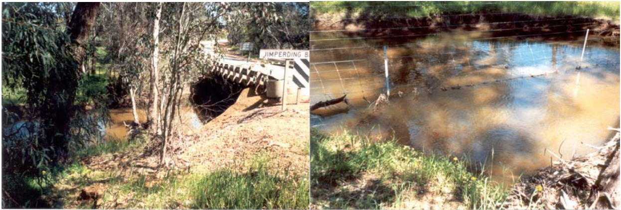
Figure 4.7a. Photos of Site 7.
