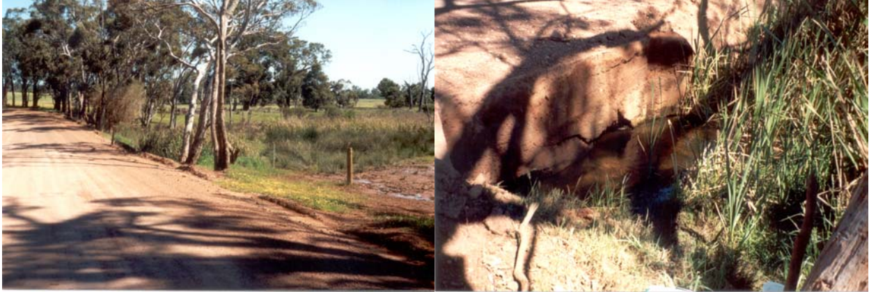
Figure 4.1a. Photos of Site 1.
